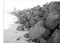
Seawall at Warilla
